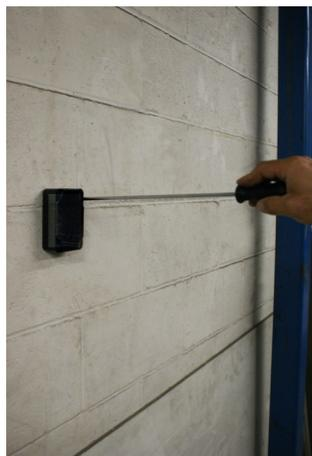
*Mount black case onto wall using appropriate mounting screws for wall conditions*
