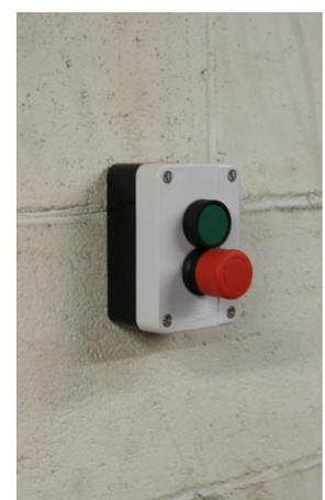
*Push button should be mounted as seen here (green button on top, red on bottom).*
