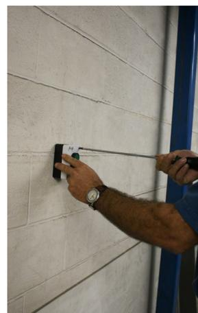
*Re-assemble the push button cover after completing wiring from enclosure.*
