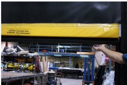
**→IF:** The Red LED light is “ON” – this indicates the impact sensor was activated. (hit by lateral/frontal movement seen here)
